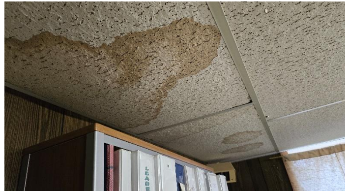
12. Basement main area ceiling water damage
