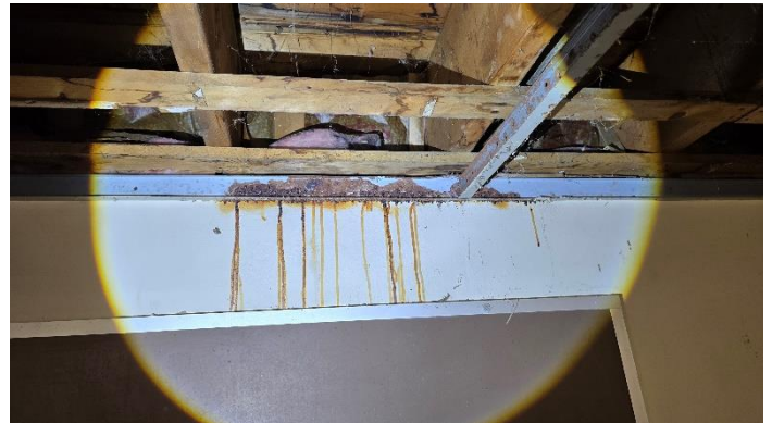
10. More water damage in the basement
