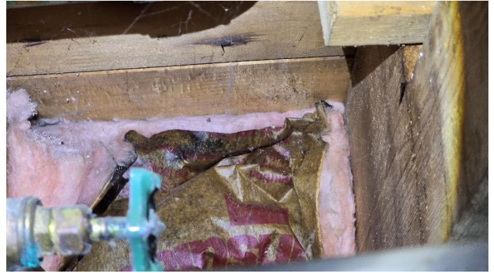
8. Basement insulation with mold
